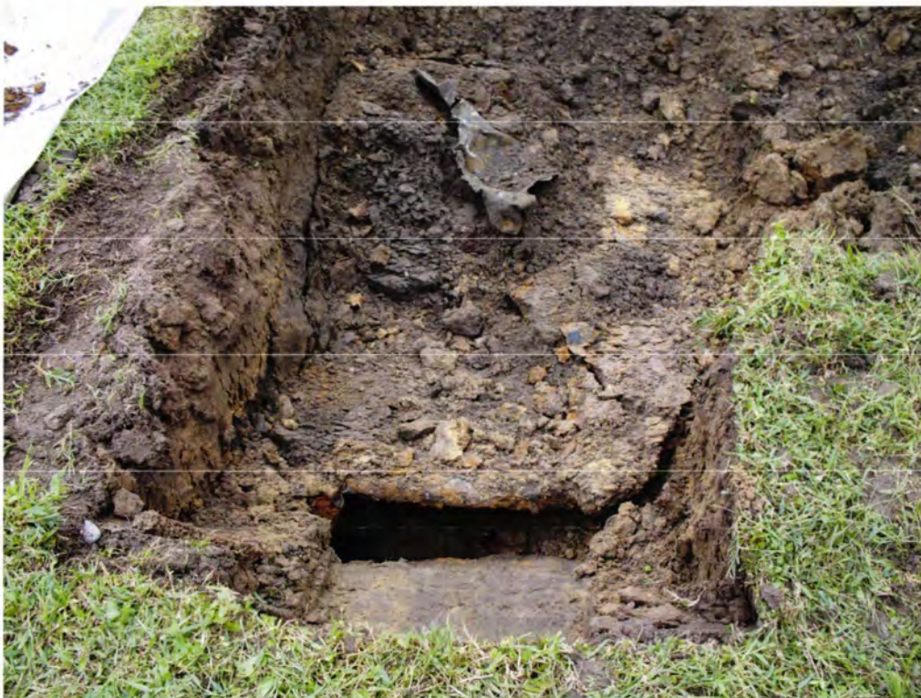
Picture 6: Excavation of UST 458Elderberry-4 in progress.
